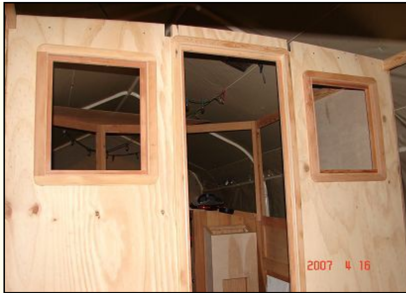
The back wall is installed.
