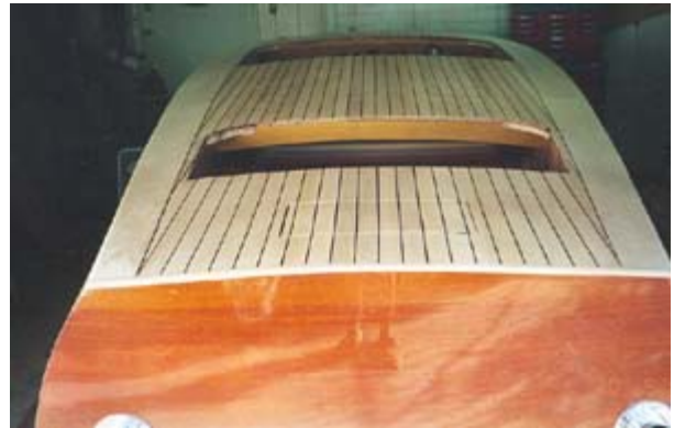
Fig. 12 thru Fig. 15 (above & below) - Authentic decking appearance is done with mahogany ply or veneer overlaid on the plywood subdeck and bonded with epoxy glue. A builder can display a lot of creativity in this area with wood staining, seam caulking, hardware placement, etc.
