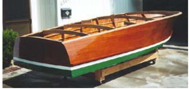
Fig. 6 - Completed hull has been removed from jig and righted for the balance of construction. John rigged up a dolly here, but you could also use the boat's trailer at this point. We have BOAT TRAILER PLANS that you can use to build your own.
