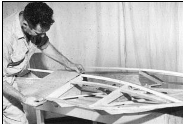
Fig. 8: Progressively checking the fairing with a scrap of plywood will help to insure that the members are properly faired for the decking.
